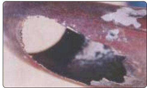
Fig. 1. Metal Erosion in U-bend.
